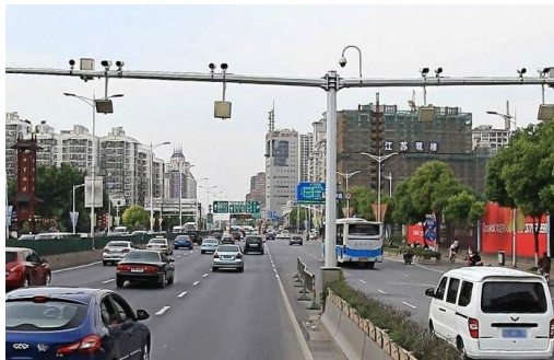
Fig.1 photo of one station
